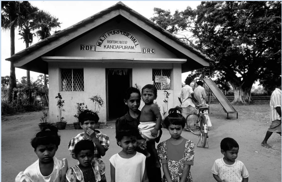
Multipurpose Hall in Sri Lankan village. Photo by Dominic Sansoni, courtesy of the World Bank Photo Library.
