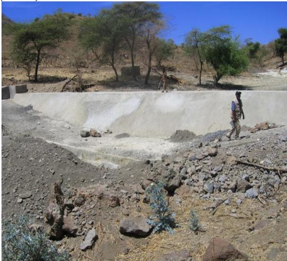
**d. Second structure constructed under another program to prevent silting of dam constructed under EDRP (above)**
