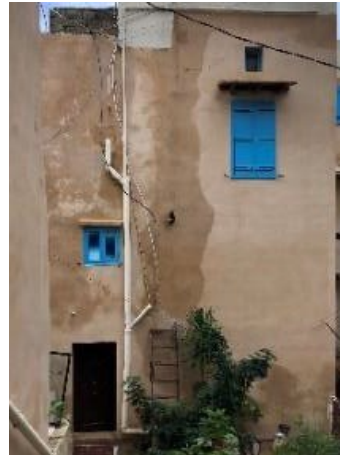
Figure 3.2. Water Leaks through CHUD-Installed Works
