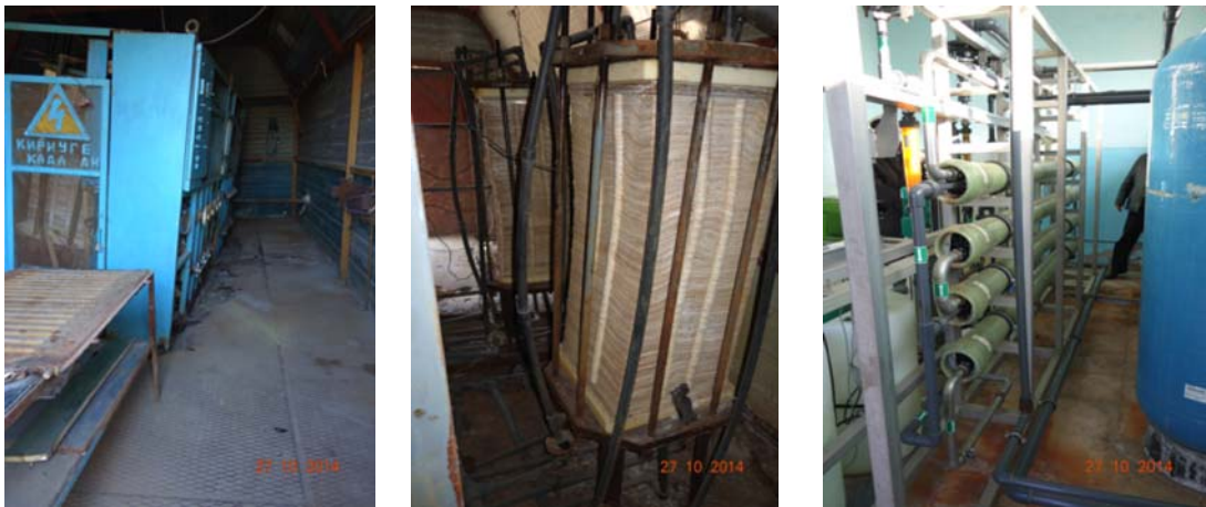
Figure 1: Worn-out small-scale desalination plants (left) were replaced (right)
