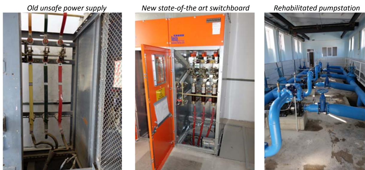
Figure 7: Rehabilitation of pumping equipment financed by the Swiss Grant
