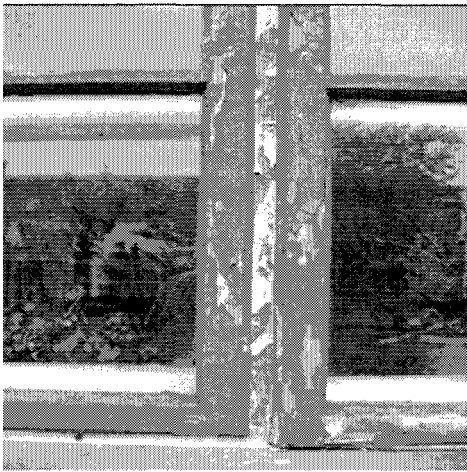
Figure 3.6: without primer, paint on windows peels fast
