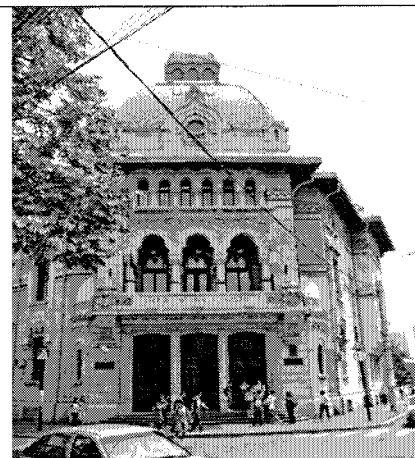
Figure 2.1: Refurbished monument school
