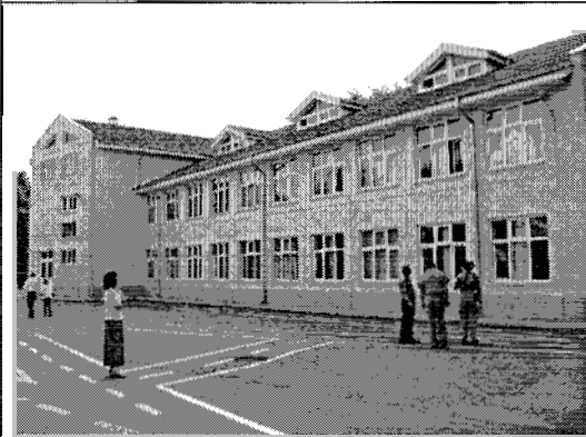
Figure 2.2: A large school rebuilt on the site of an earlier one
