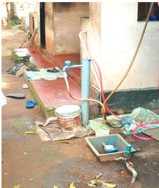
Figure 3. A Typical Household Metered Water Connection in Kerala
