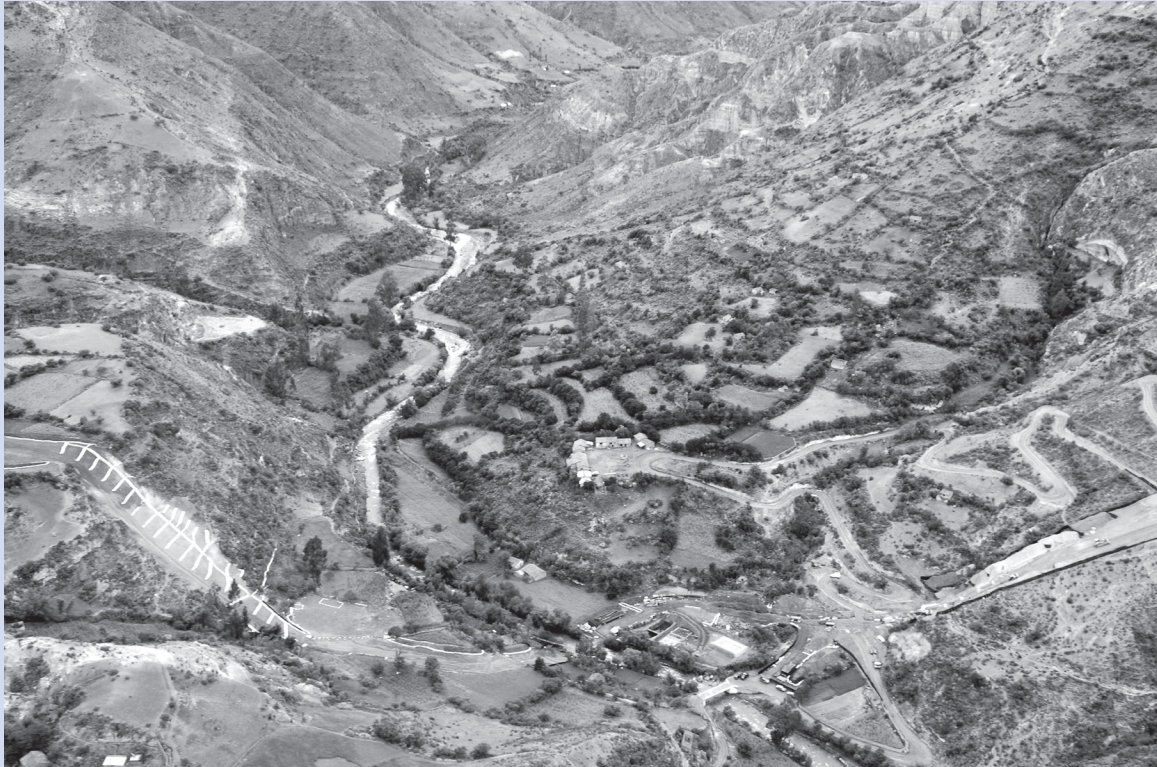
Construction of a pipeline in Peru. Photo courtesy of Jouni Martti Eerikainen.
