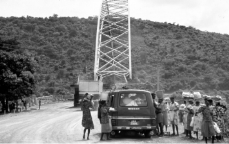
A bridge in Ghana. Photo courtesy of World Bank Photo Library.
